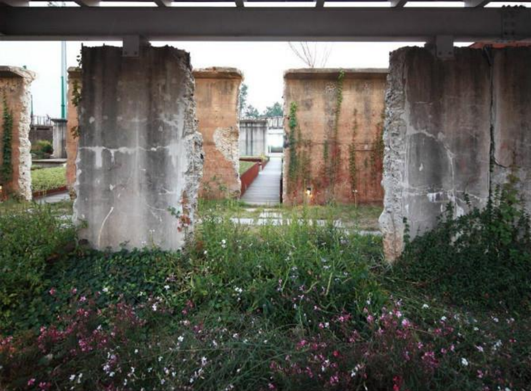
PA-526-09 Detailed view of reused industrial walls. The walls of the water purification chambers, which were part of the former industrial facilities, not only act as a basic structure of the Floating Promenade but provides a private landscape and an original natural spectacle, through sharp contrast and native plants. ( Aster koraiensis ,
