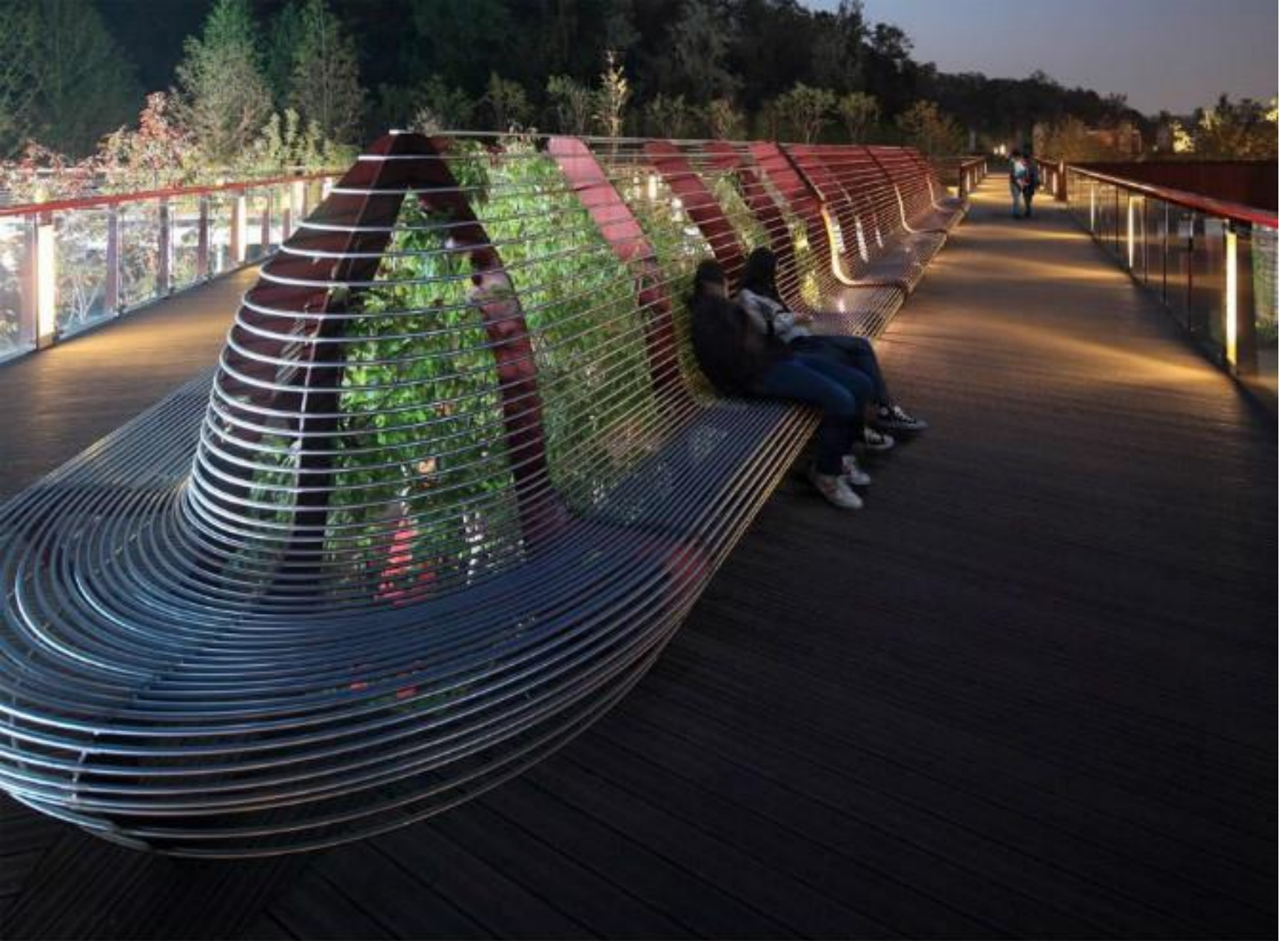
PA-526-11 Night view of Floating Promenade. Bench with interconnected backrest functioning as both fence and guardrail provides ample seating and expansive views for park users.
