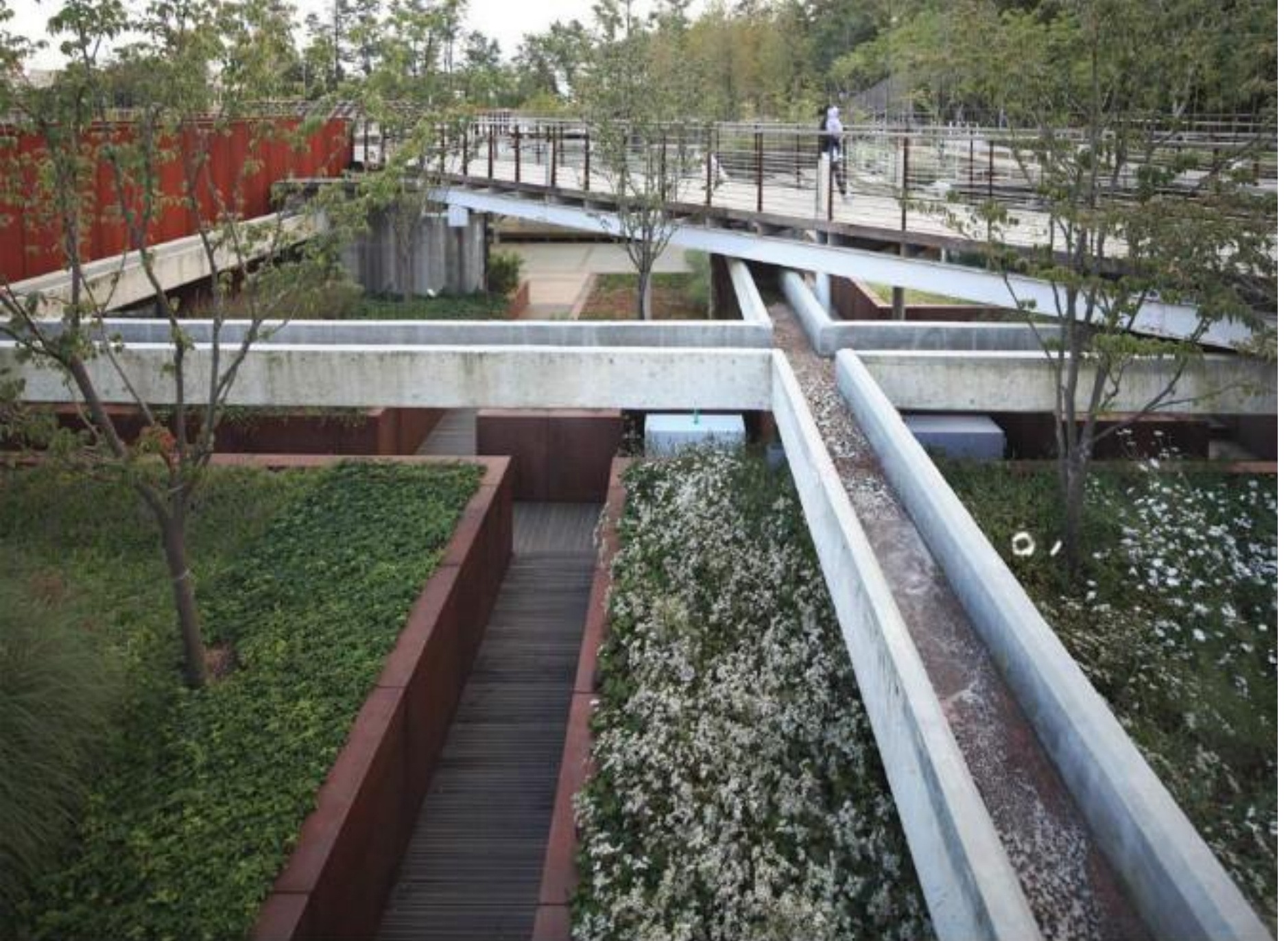
PA-526-05 Floating Promenade and purification canal above the garden path. Three differing layers forming a reiterating sight offers the visitors a plentiful experience of space. The waterways activating former constructions creates an eco system that connects the purified water to the lake.
